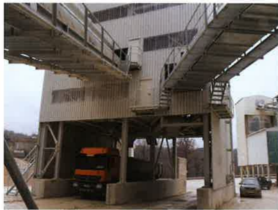
Fig. 2: Loading and transportation in the ballast works
